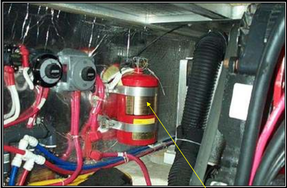
Engine Space – Electrical Systems & Fire Suppression
