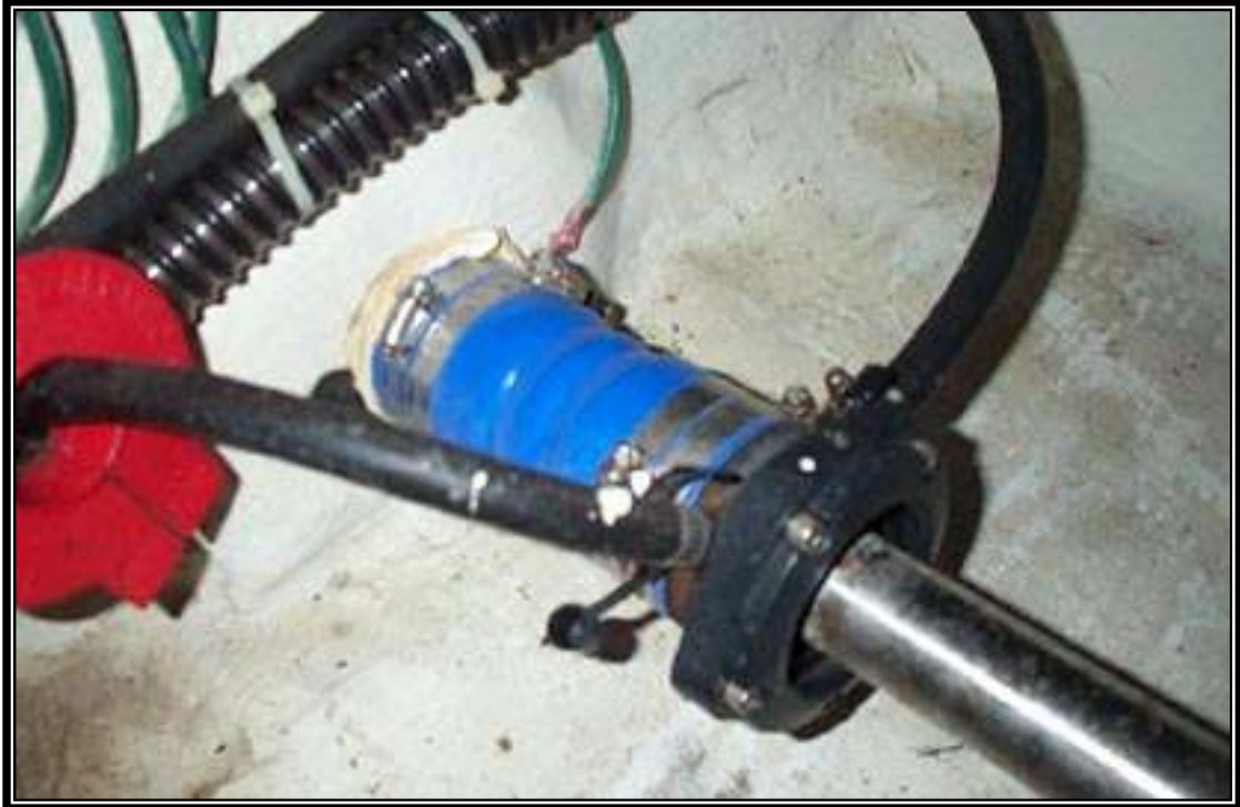
Port Propeller Shaft Log
