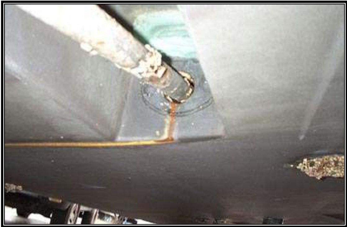
Starboard Propeller Shaft – Note Discolored Drippage
