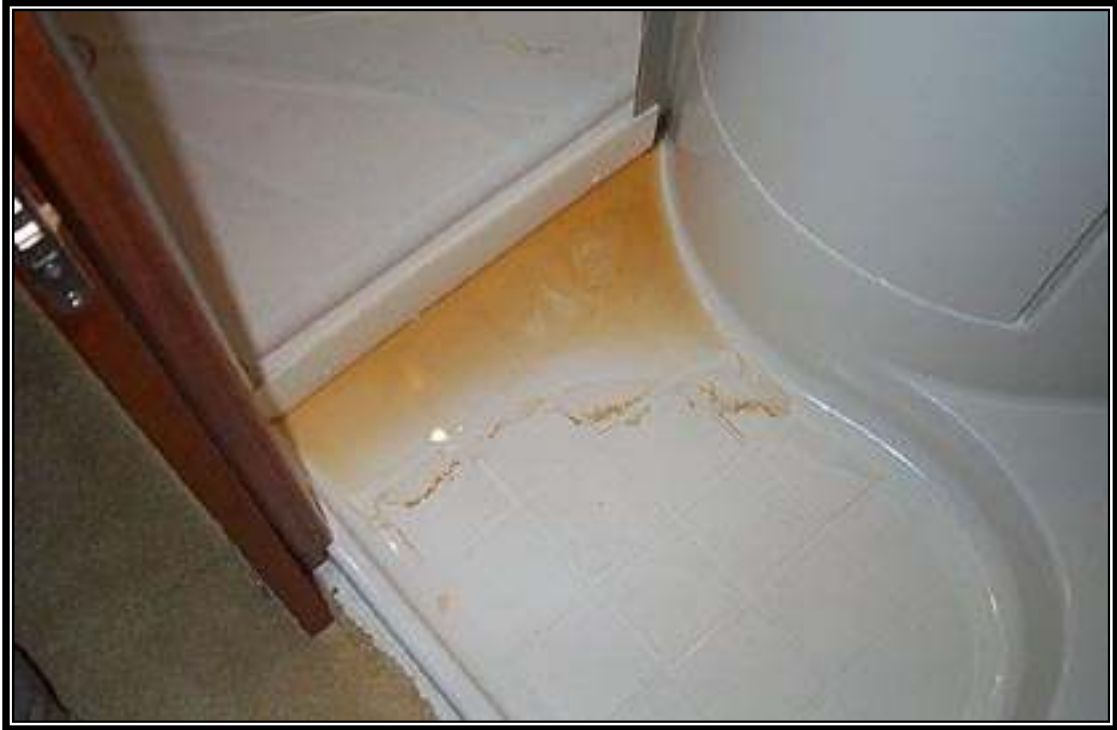
Ice in Aft Stateroom Head Area
