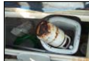
Leaking Propane Tank
